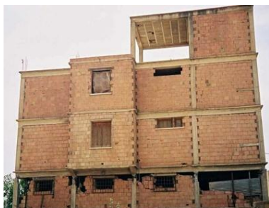
Figure 1.1 Multi storeyed frame with infill
